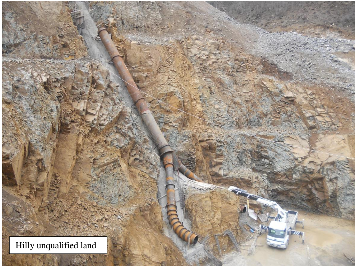
Annex 7.2: Penstock (During Construction)
