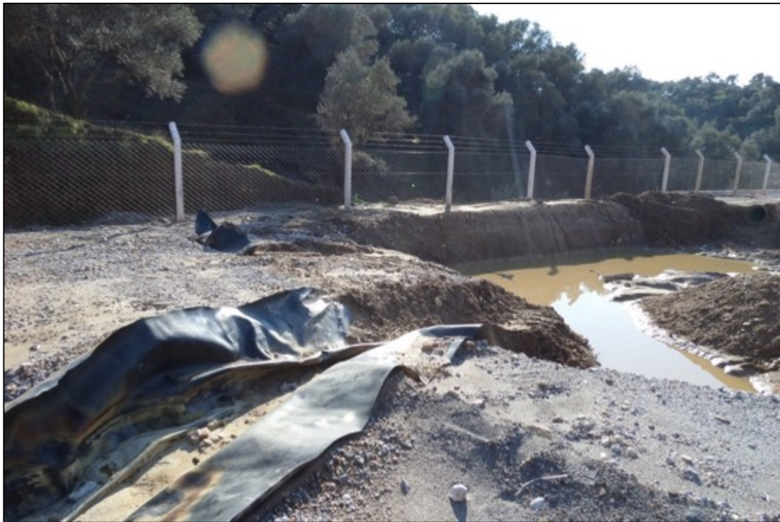
Photo 7-1. Mud Pits Lined with Geomembrane
