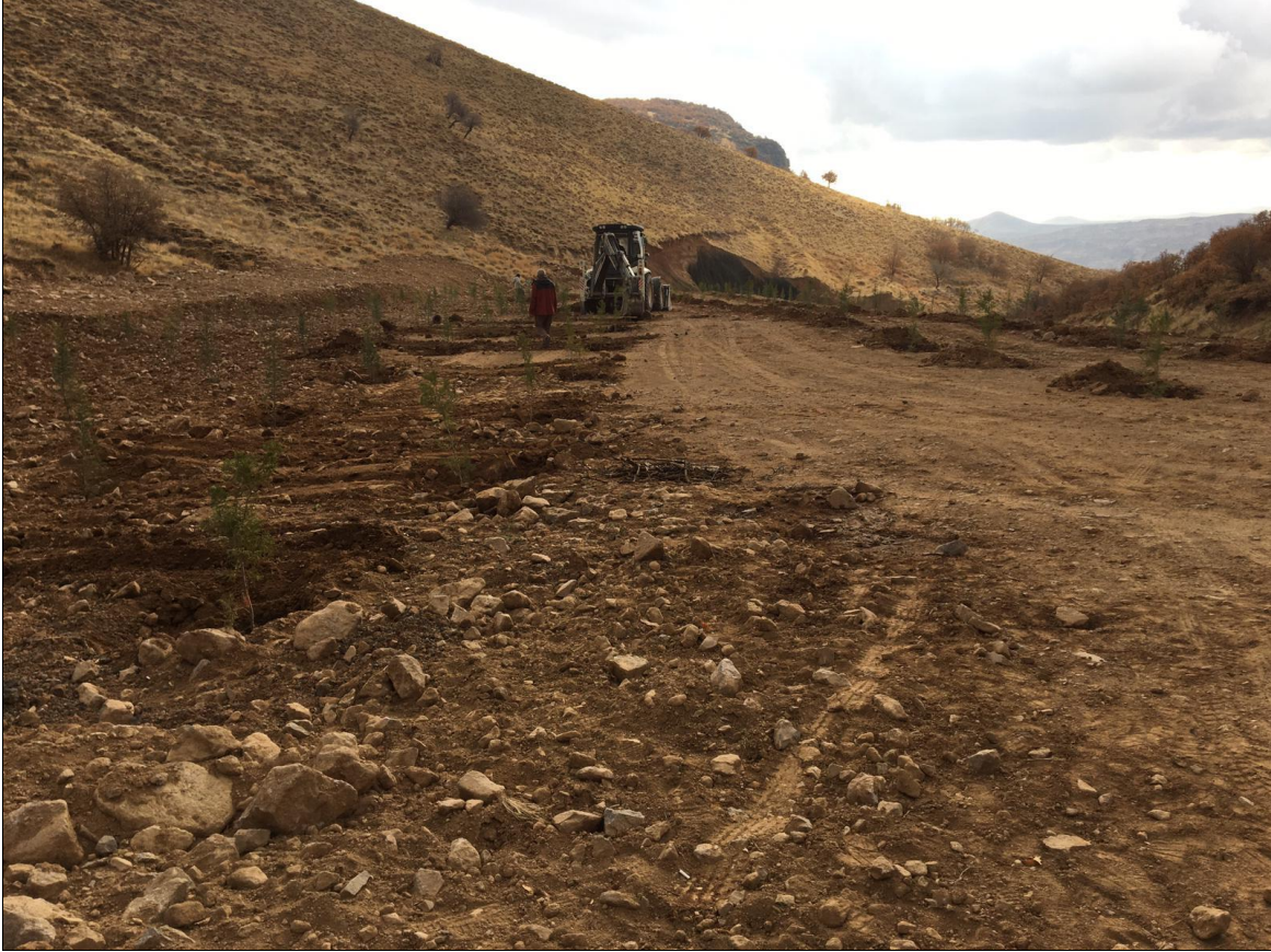
Figure 32. The Figure Shows Planted Area
