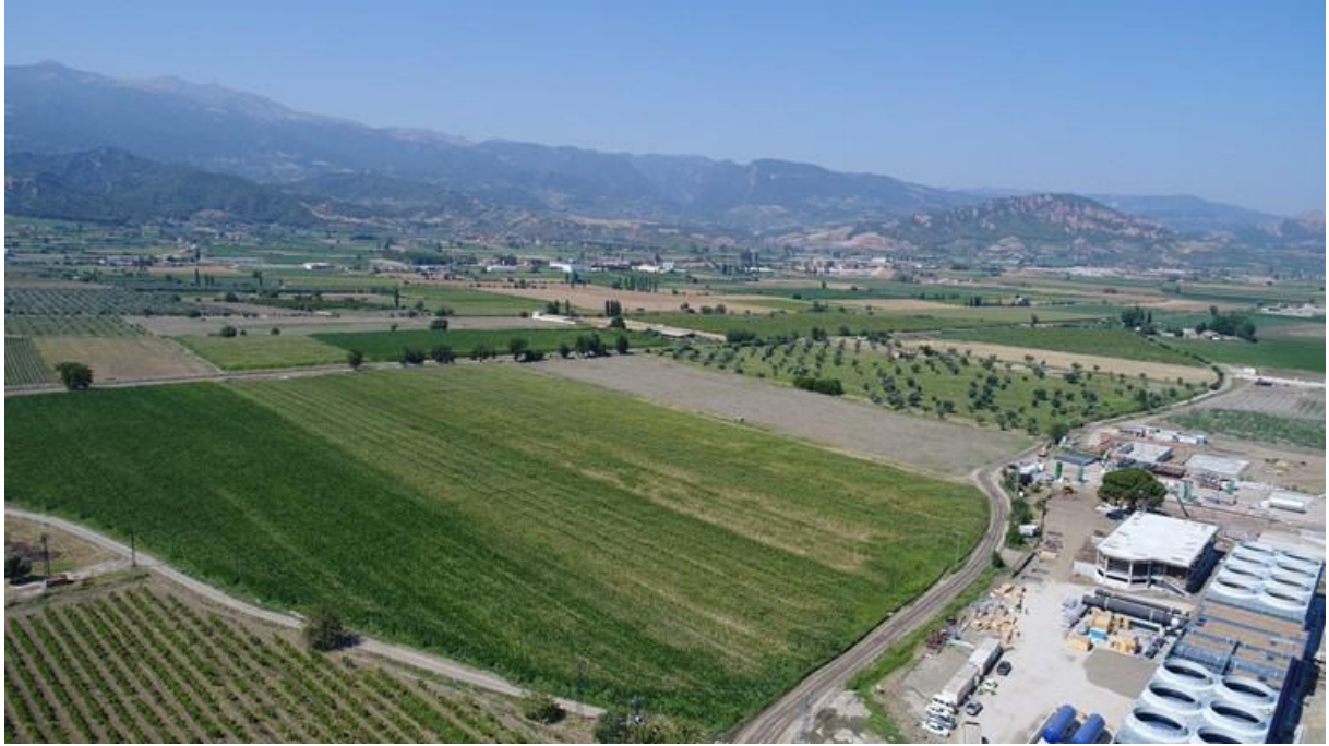
Photo 5-3. Agricultural and Residential Areas Around Power Plant
